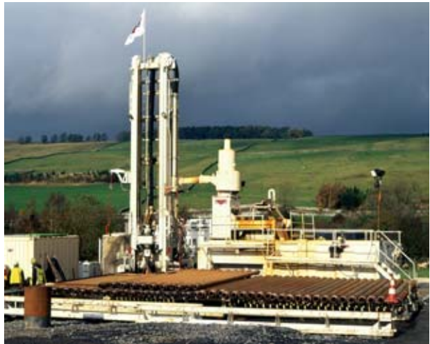
East Gate drilling rig working on the borehole for the new geothermal energy project
