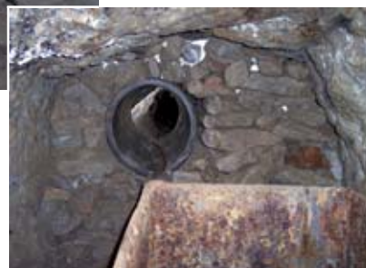
Below: View of the 'inbye' side of the tube with part of the end tipping truck (featured in Journal 9) in the foreground.
