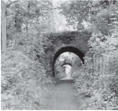
The ironstone cartway bridge & the Coalport Branch Railway Bridge over Gypsy Lane, Aug. 1968 (I.J.Brown)
