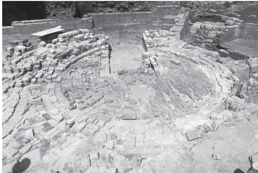
Base of Haystack boiler at Blists Hill 'Upper' Mine, stoking area and grate were in the rectangular section at top middle of picture.
