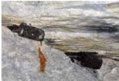
Above: Two metal wedges still in situ - these were driven in to separate one block of stone from another.
